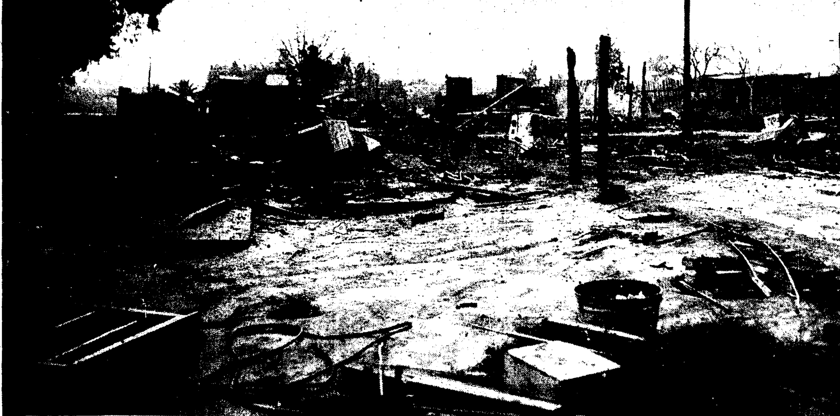
CHARRED RUINS—Ashes and charred ruins remain after blaze which destroyed seven houses along Southworth St. at the edge of Montebello, and left more than a score of persons homeless. The fire spread quickly, menacing dozens of other small dwellings.
